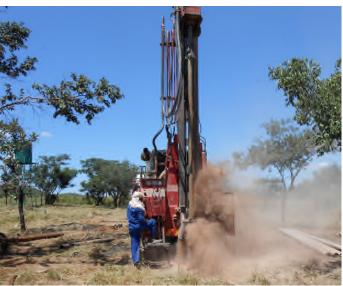
Pictured above is the drilling rig beginning to drill the hole. Pictured to the right is the result (water coming up out of the hole from 90 meters below). This bore hole will provide drinking water to our Student and Senior Staff houses and water for the student gardens.
