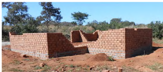
Student house under construction
