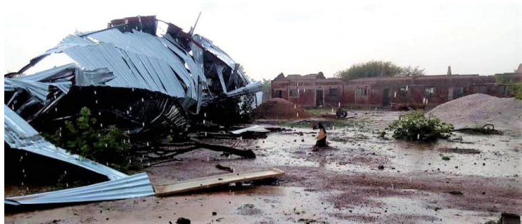
New classroom wing after the storm
